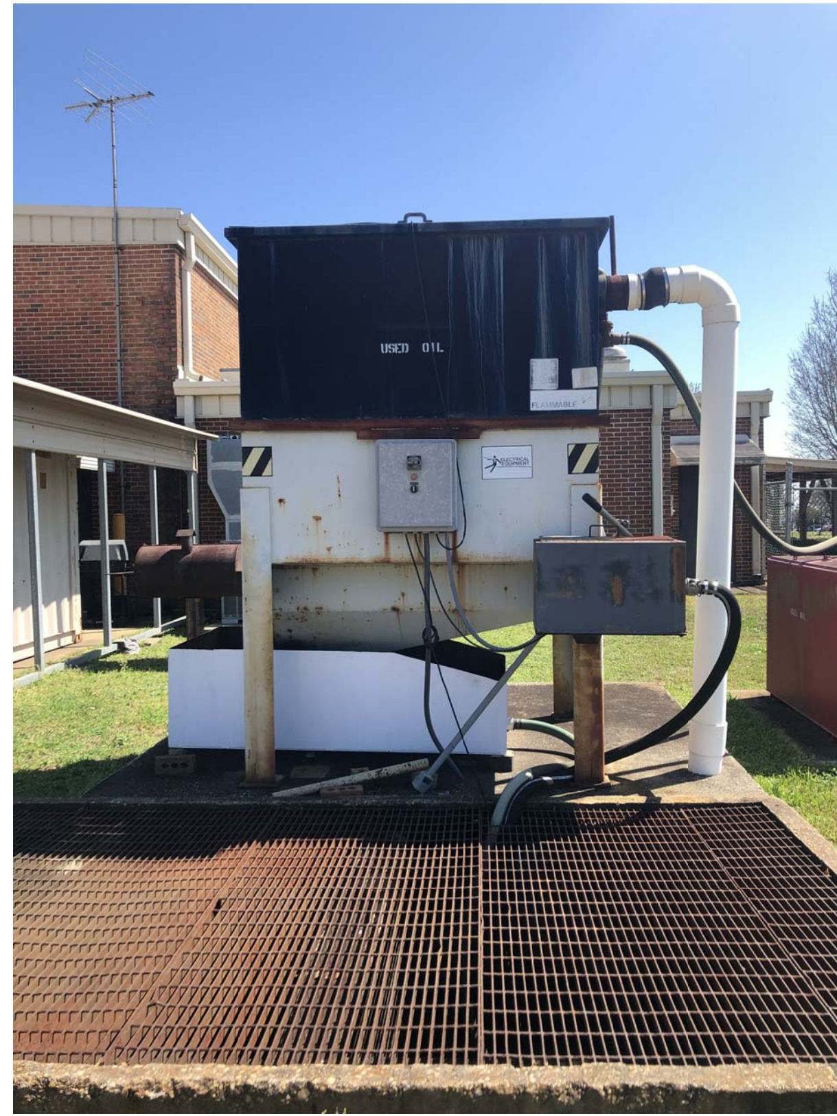
EXISTING OIL-WATER SEPARATOR
