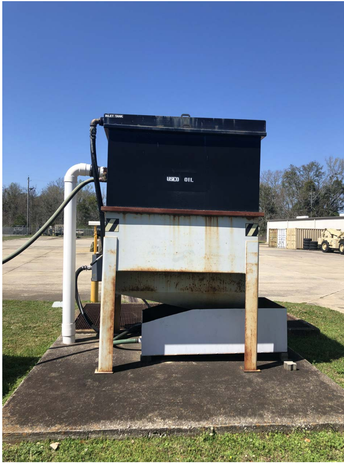
EXISTING OIL-WATER SEPARATOR
