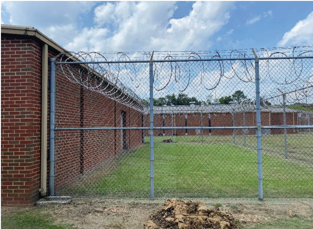
Figure 1: Typical conditions near B-01 facing north
