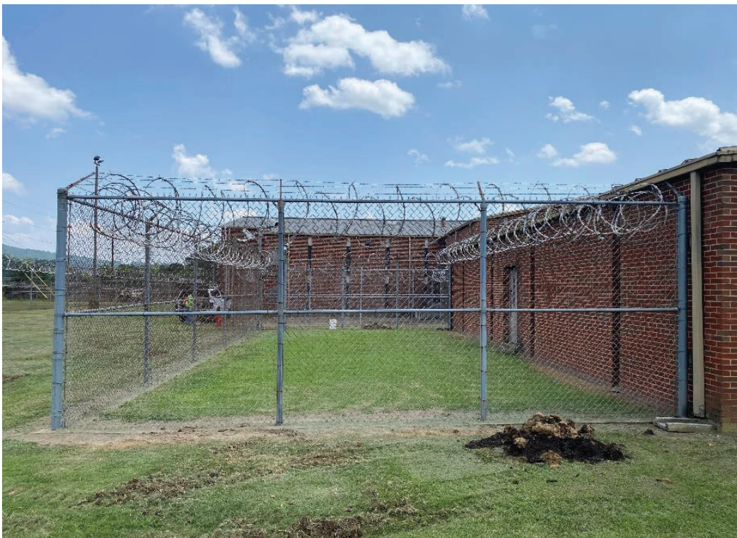
Figure 2: Typical conditions near B-02 facing south
