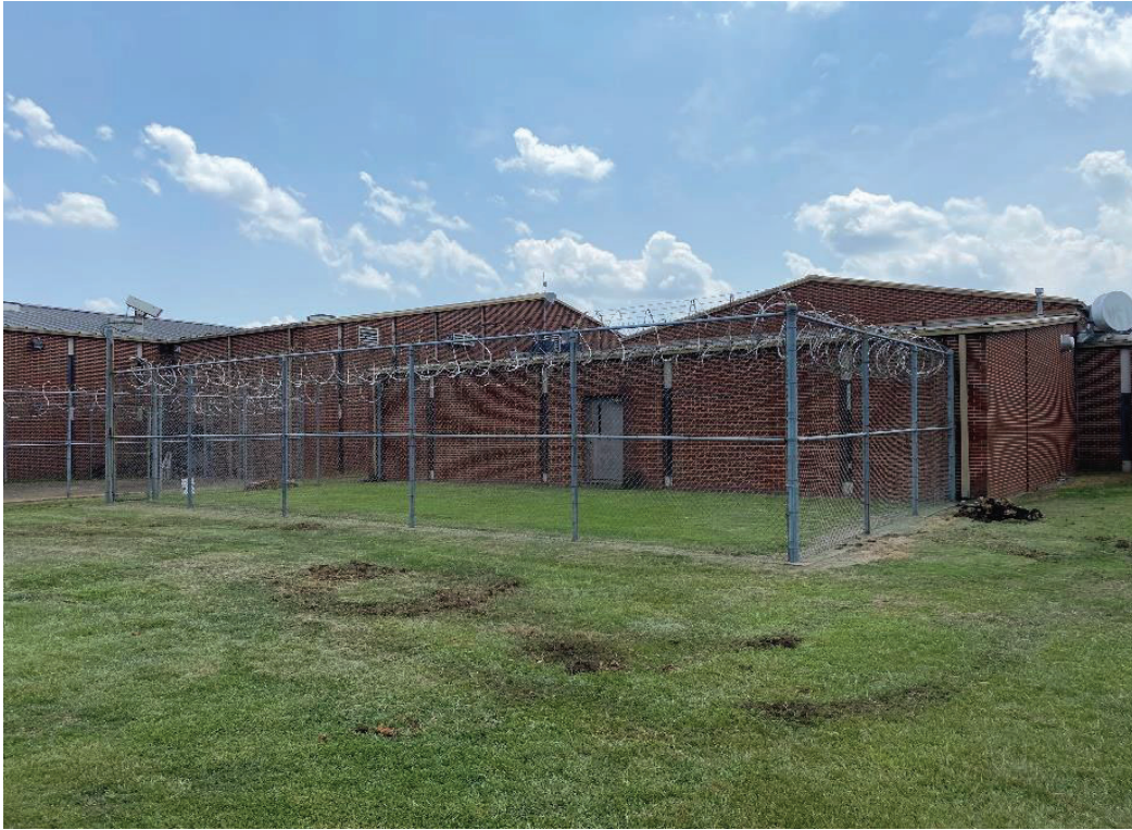
Figure 3: Typical conditions near B-05 facing southwest
