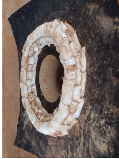
Figure IP-4 Sand Bag Inlet Protection Installation.
