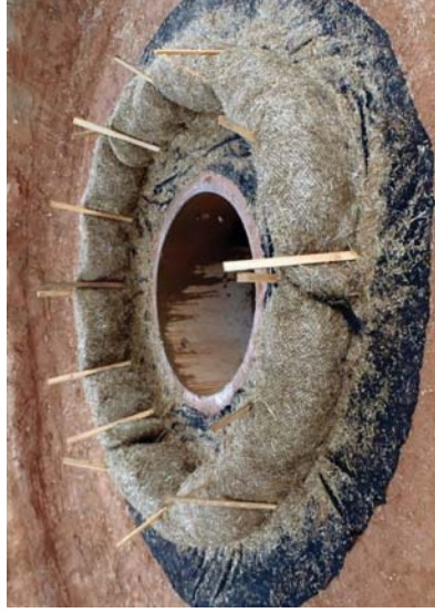
Figure IP-5 Wattle Inlet Protection Installation.
