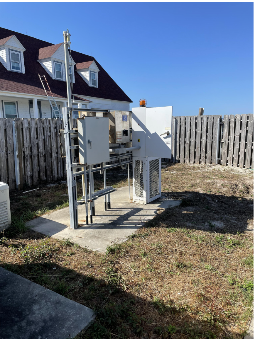
6 PANEL, SPD, PUMP CONTROLLER E301
