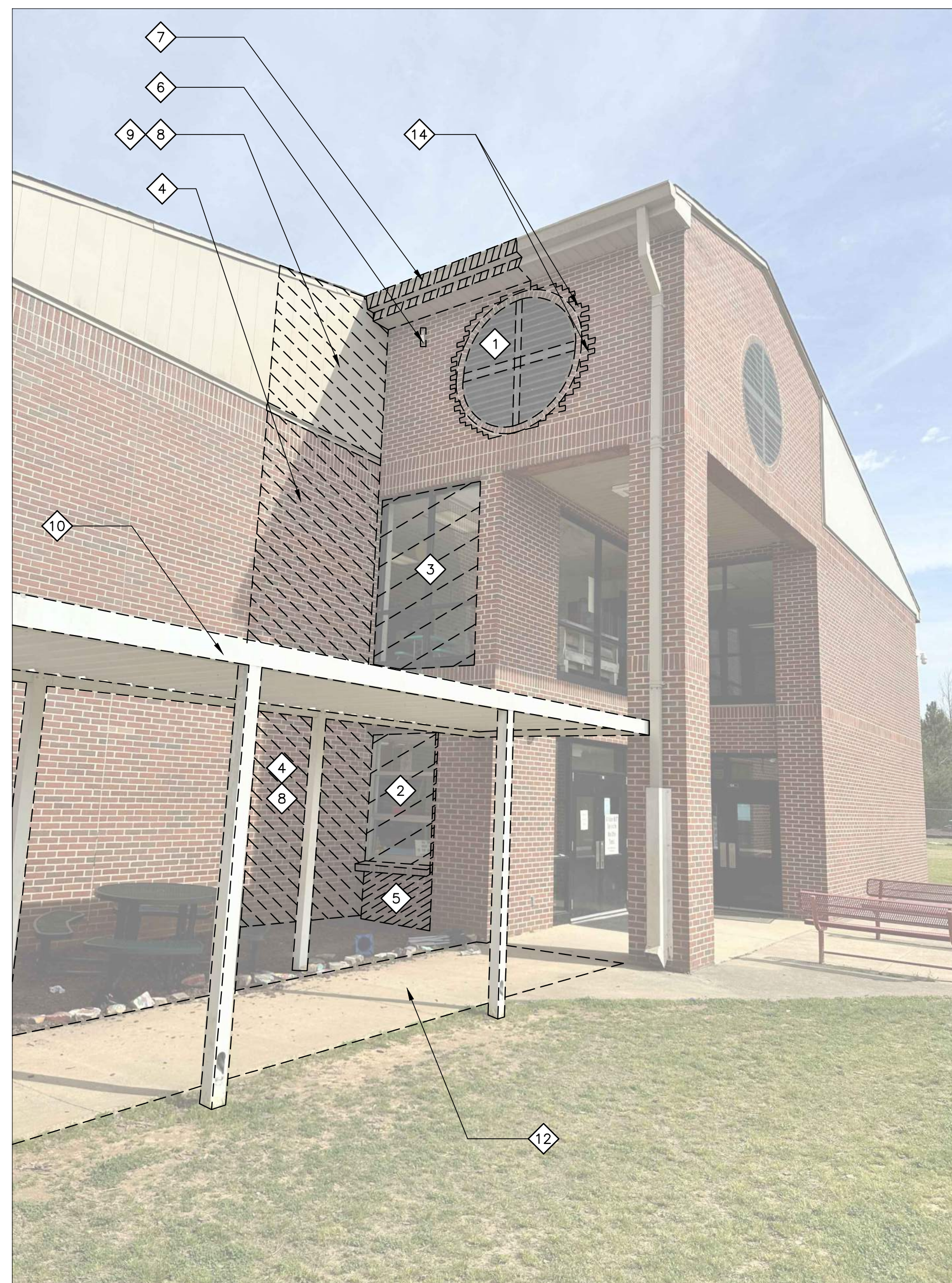
B DEMOLITION PHOTO
