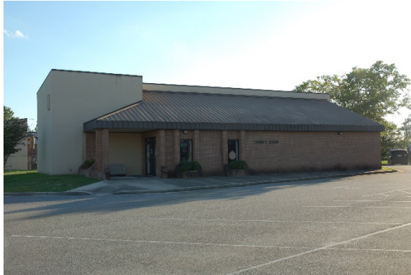
4-9d Furniture Store in the Admin/Community/Retail Area.
