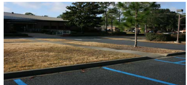
3-6a Sidewalks leading from parking lot to the main building across the street.
