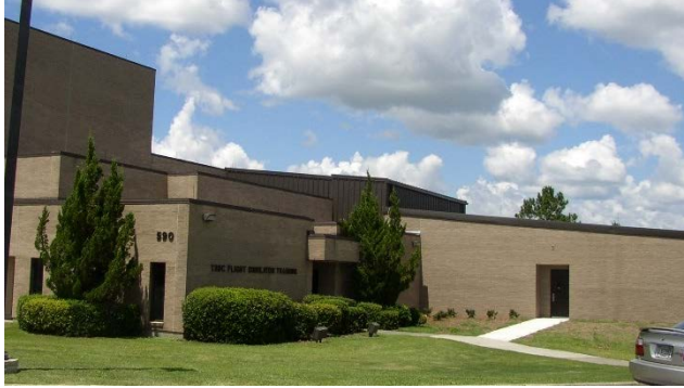
4-2b BLDG 590 addition
