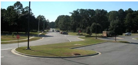
3-8e Parking design at enlisted dormitories incorporates landscaping to define circulation.
