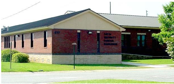
4-9b Examples of acceptable brick and CMU usage on the 23d Security Forces Squadron facility.
