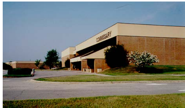
4-10d Brick and mortar colors of the existing Community Center buildings set the standard for exterior wall materials in the Admin/Community visual area.
