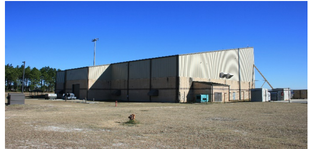
2.3c Wash Rack in C-130 Building 642
