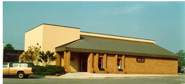
4-10c Future buildings in the Admin/Community Area will match the brown brick and dark bronze metal roof of the Thrift Store.
