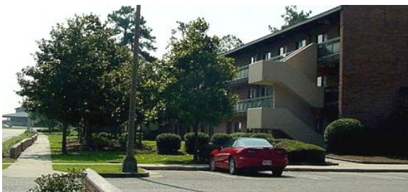
3-8f Use of both trees and shrubs provides shade and screens parking from the street.
