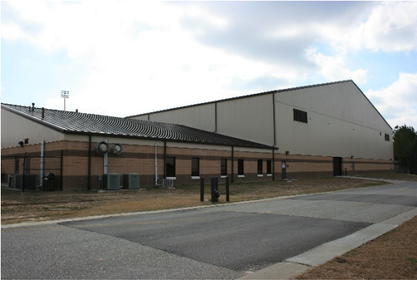
2.3e Building 730. Downspout color matches roof color.
