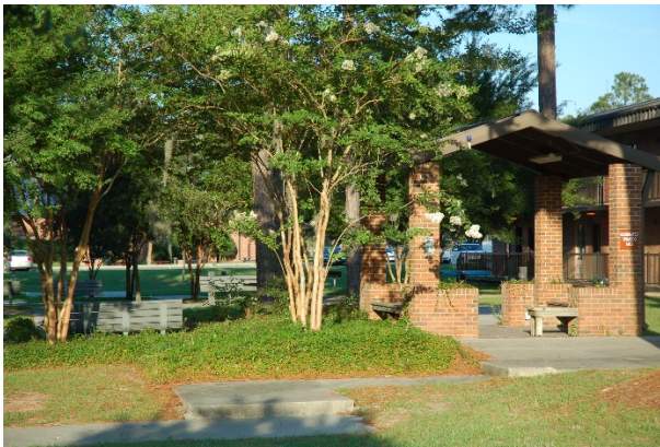
4-14c Picnic shelter in the 300 area dormitories area.
