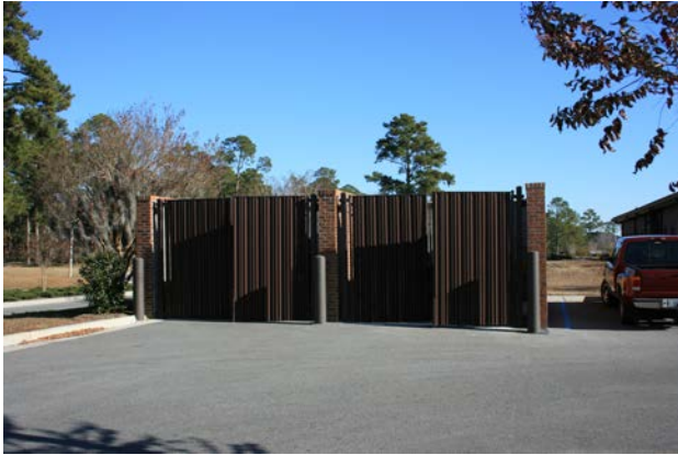
3-7e Dumpster enclosure matches masonry of nearby buildings.
