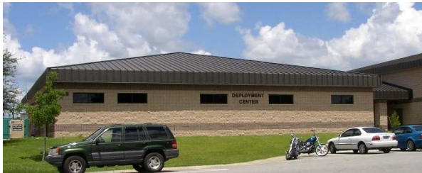
4-9c Examples of acceptable CMU usage on the Deployment center facility.
