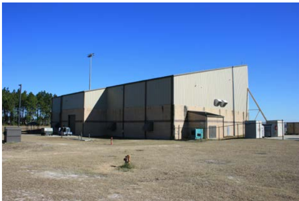
4-5c C-130 Wash Rack: Simple, functional form
