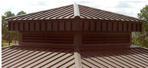
4-6d Roof ventilation.
