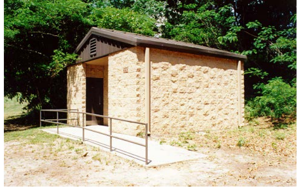
2.5g Restroom facility
