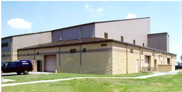
4-5b Sloped roofs and additive forms give human scale to large building masses.
