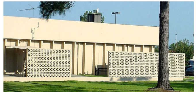
4-4a Utility equipment and trash receptacles located and screened appropriately.
