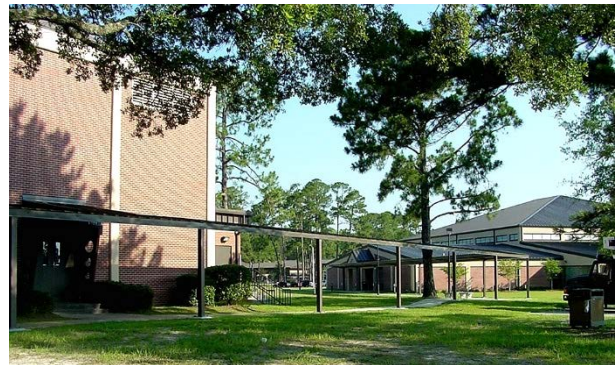
3-7b Covered walkway connecting the new gymnasium building to the old gym.
