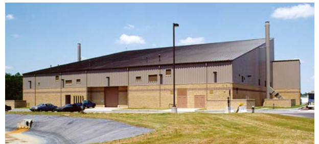
2.3d Buildings in the C-130 Complex use concrete masonry base with beige metal wall panels above, and dark bronze metal roofing.
