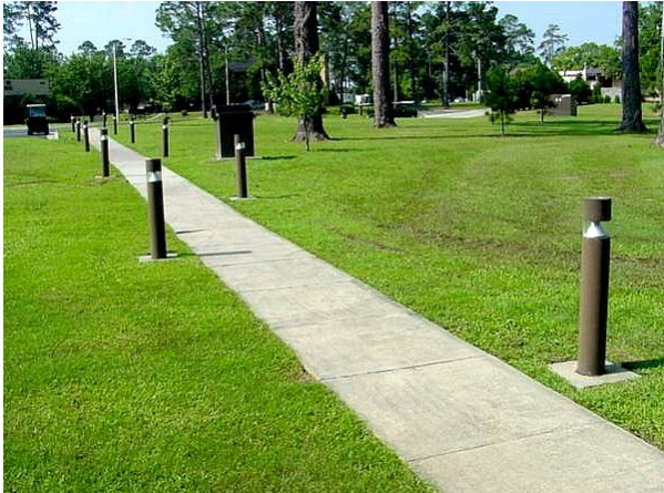
3.7a Bollard lighting fixtures in Unaccompanied Housing Area.
