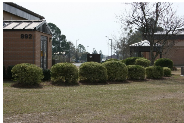
3-8h Landscaping to screen transformers and equipment.
