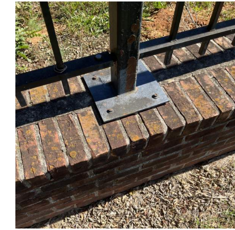
TYPICAL IRON POST CONNECTION AT FENCE
