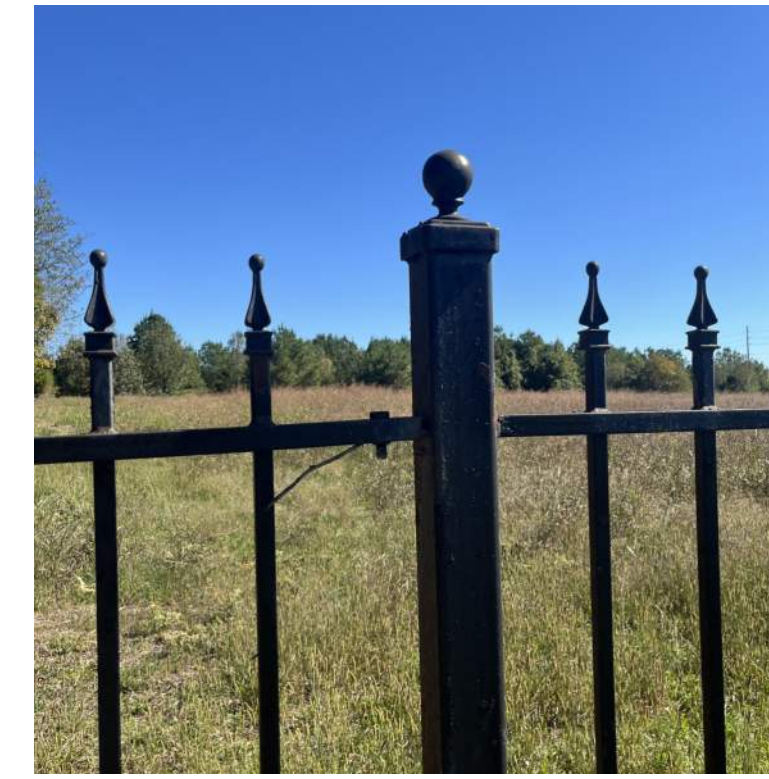
EXISTING FINIALS AND POST CAP AT IRON FENCE
