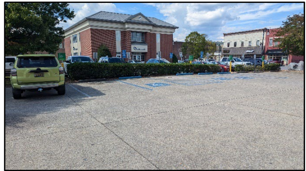
Looking North Towards 2-story Building
