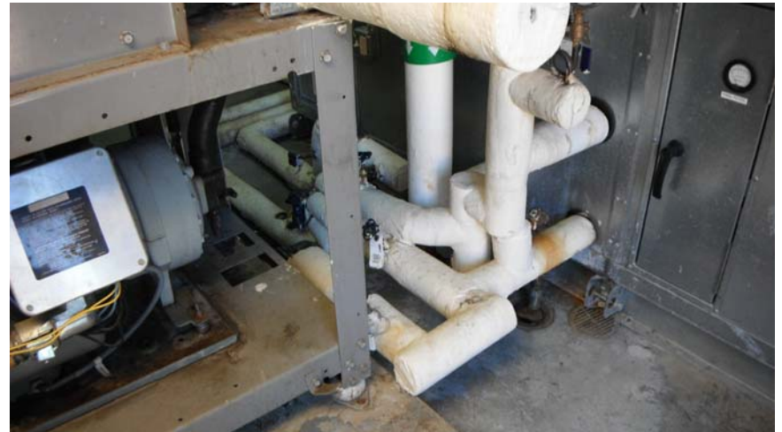
PHOTOGRAPH 4 Piping insulated with kraft-faced fiberglass insulation in mechanical room. Mastic (HA 16 – NAD) is present at raw ends and seams of this piping.
