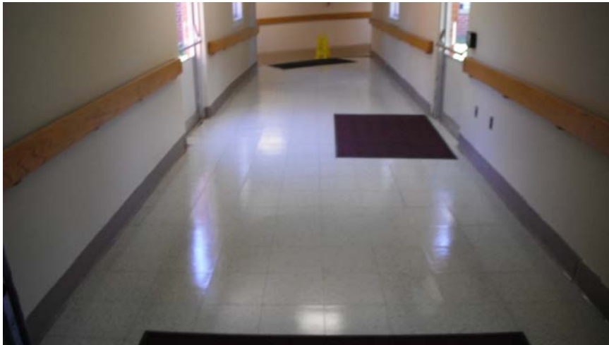
PHOTOGRAPH 2 HA 03 – ACM 12" Vinyl composition floor tile and mastic in connecting corridor to Building 1.
