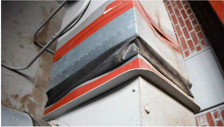
PHOTOGRAPH 5 Example of a newer, vinyl flexible duct connector in attic.
