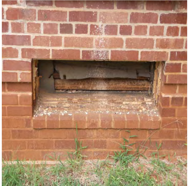
Photograph 2 Damaged/deteriorated LBP on crawlspace vent on exterior.
