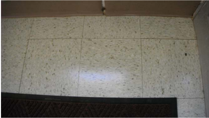
PHOTOGRAPH 1 HA 03 – ACM 12" Vinyl composition floor tile and mastic in connecting corridor to Building 1.
