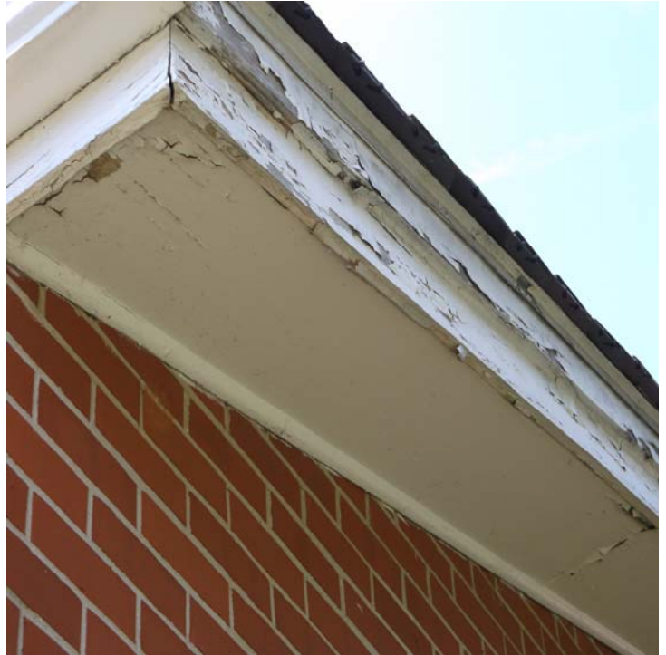
Photograph 6 Damaged / peeling LPB on wooden soffit and fascia – typical.
