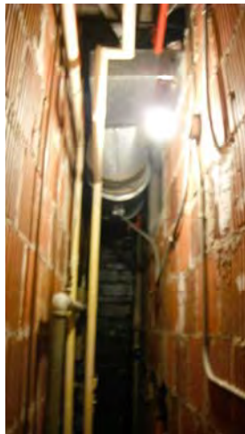
PHOTOGRAPH 6 HA 25 – ACM Flexible duct connector present in Pipe Chase 23B.
