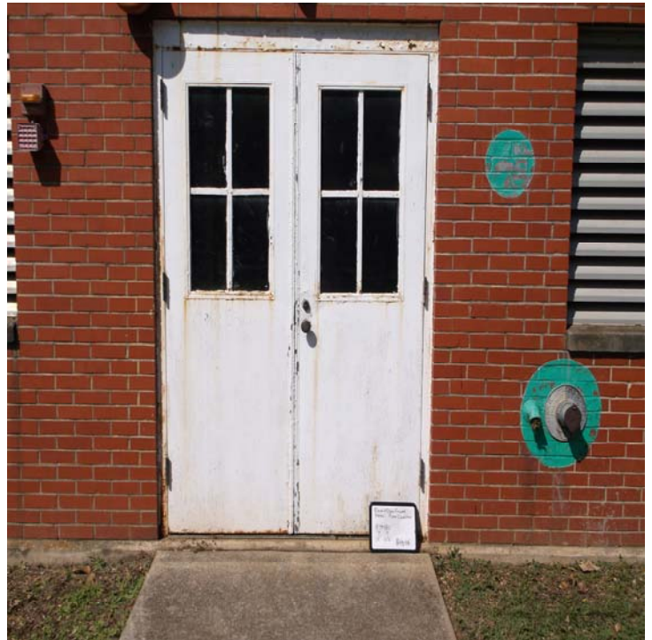
Photograph 4 Damaged LBP on metal door and frame to Room 4.
