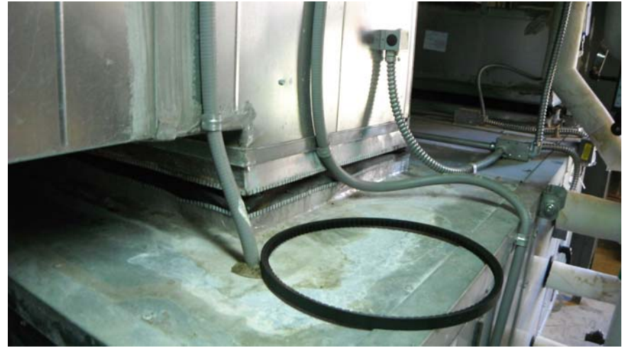
PHOTOGRAPH 3 View of rubber/vinyl flexible duct connector in mechanical room, and grey/green mastic on seams of AHU ductwork (HA 16 – NAD).
