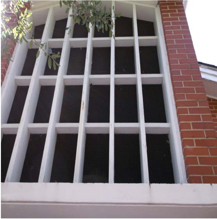
Photograph 1 Damaged LPB on wooden decorative grill.
