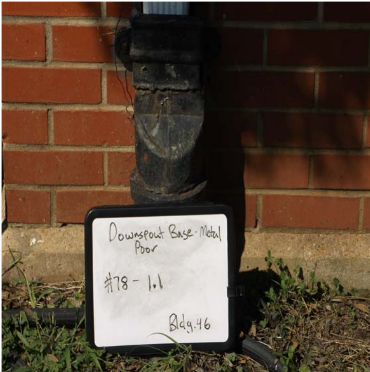
Photograph 3 Damage LBP on metal down spout base – typical.
