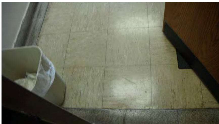
PHOTOGRAPH 2 HA 12 (ACM 12" brown VCT and mastic). Photograph taken in Room 203.
