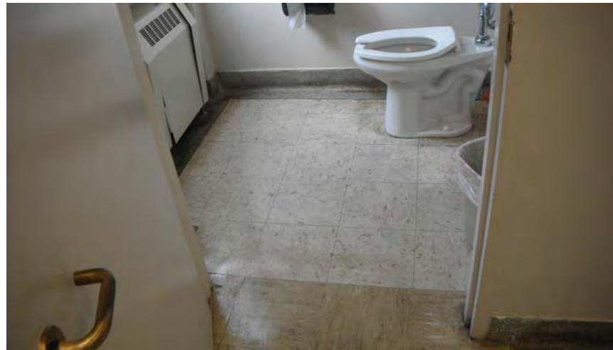
PHOTOGRAPH 3 HA 13 (ACM 12" off-white/brown VCT and mastic) in Room 203B.
