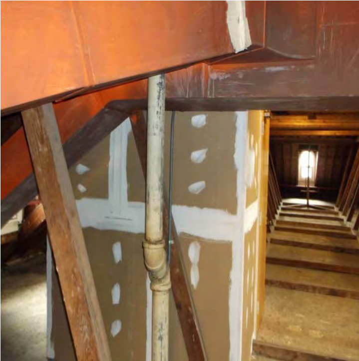
Photograph 1 Damaged LBP on metal roof drain pipe.
