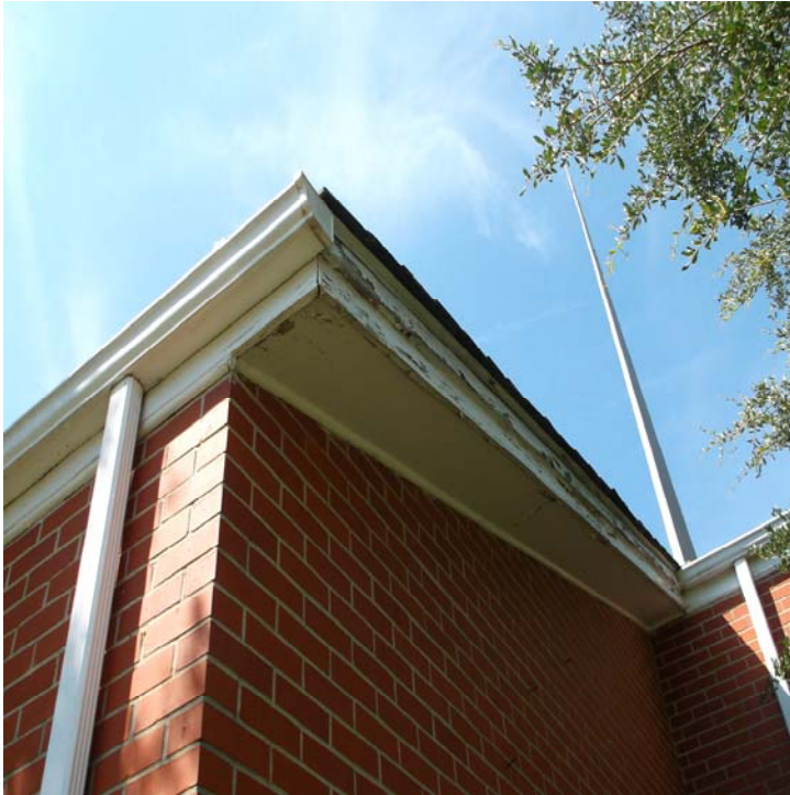
Photograph 5 Damaged / peeling LPB on wooden soffit and fascia – typical.
