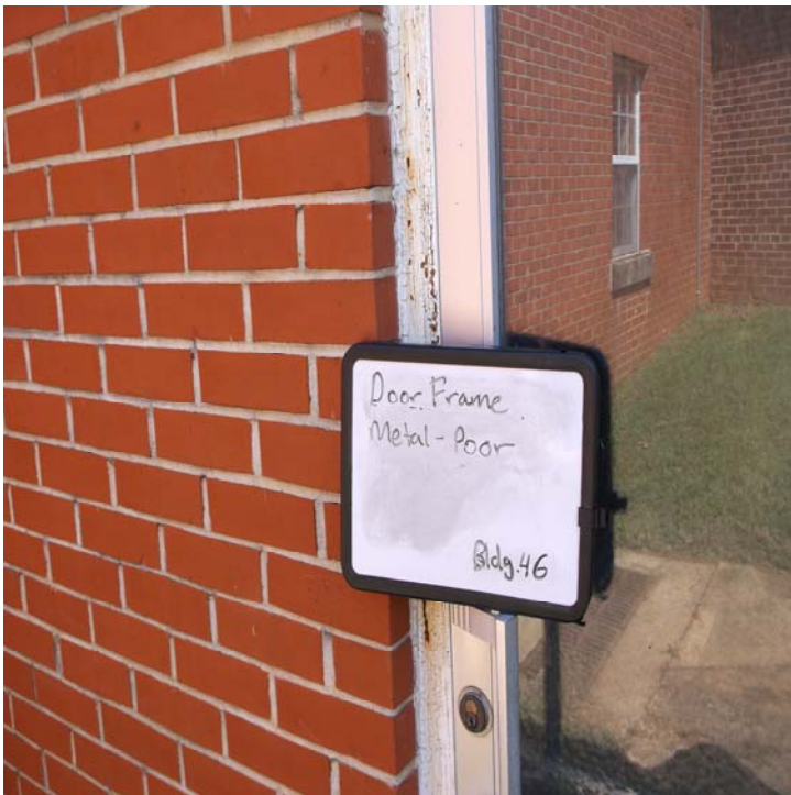
Photograph 7 Damaged / peeling LPB on exterior metal door frame – typical.
