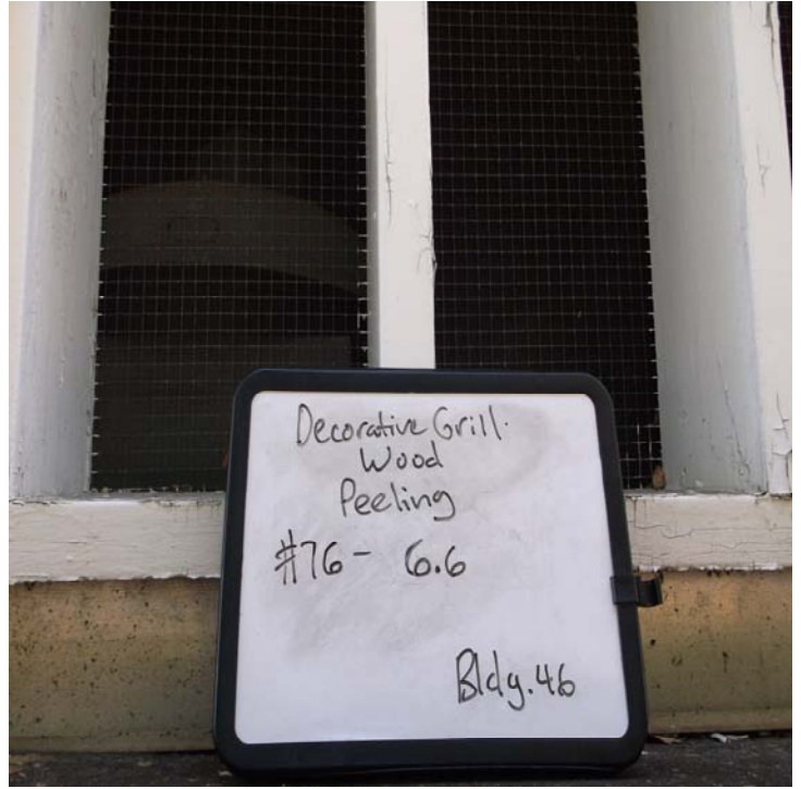
Photograph 2 Damaged / peeling LPB on wooden decorative grill.
