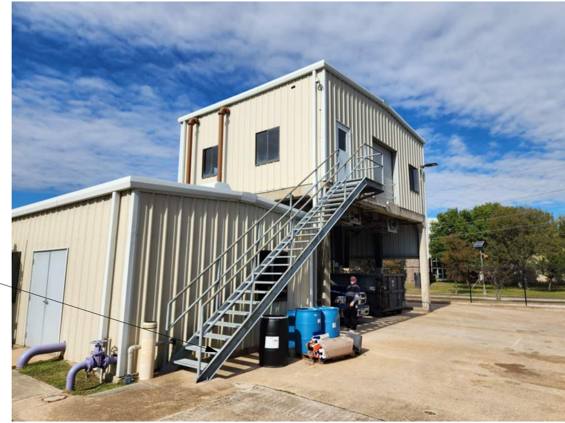
SLUDGE BELT PRESS - EAST
