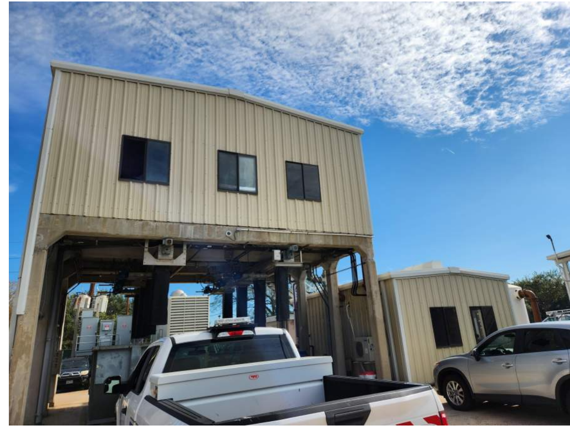
SLUDGE BELT PRESS - WEST
