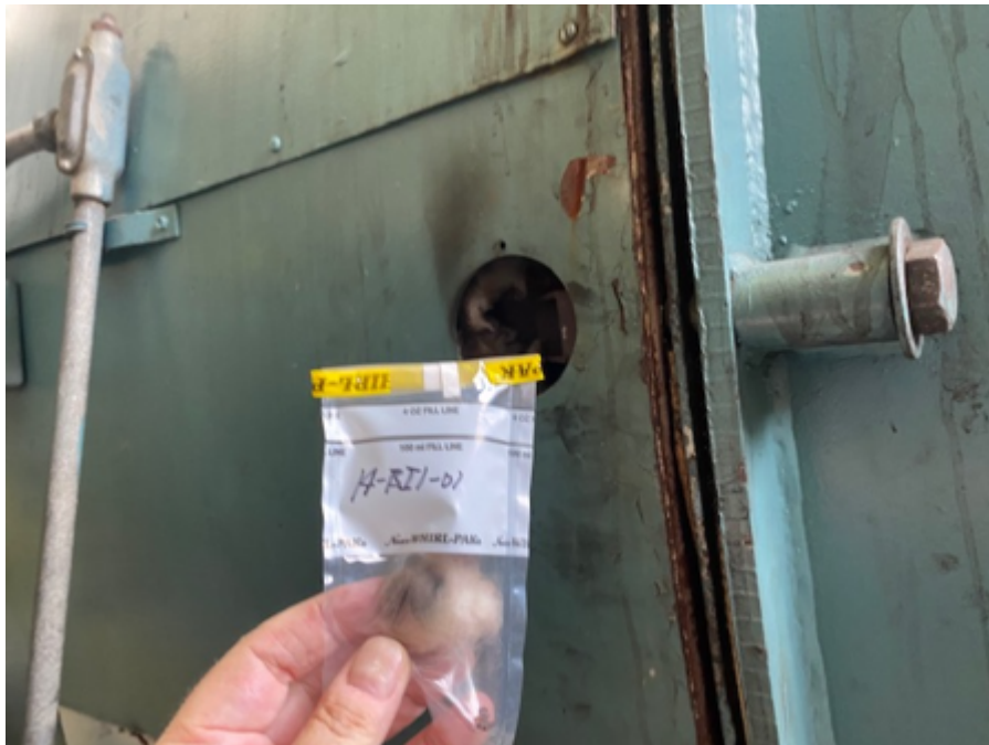
8. Boiler Insulation, Glass Fiber Type (HM #8)
