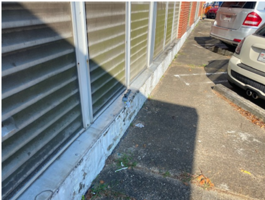
7. White Paint on Exterior Concrete Wall, Building 14, Exterior (Sample #14-PC-07)
