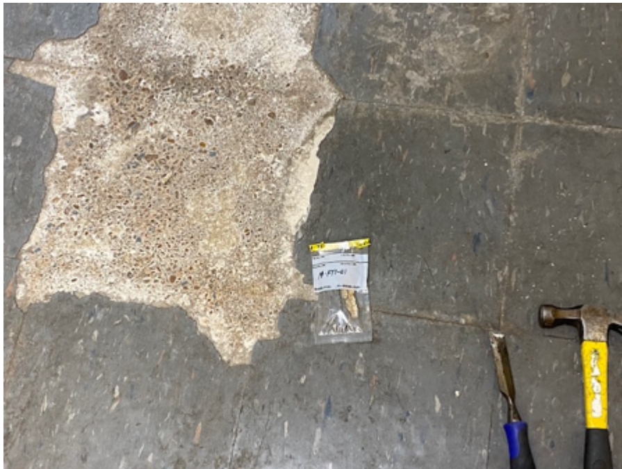
4. 12" X 12" Gray, Floor Tile and Associated Mastics, Glues & Adhesives (HM #4)
