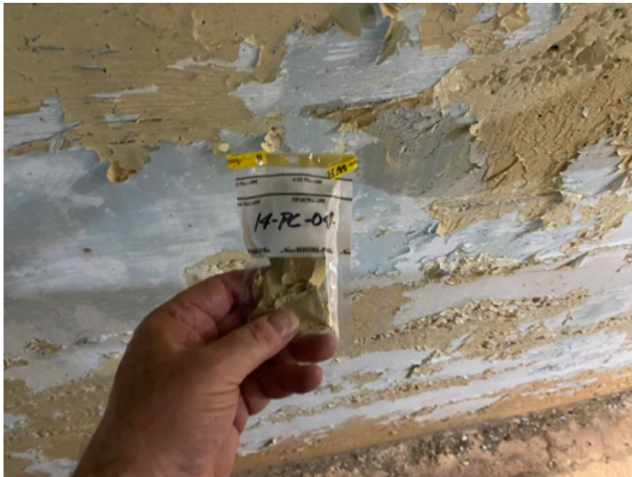
4. Beige/Yellow Paint on Concrete Wall, Building 14, Pipe Tunnel Walls (Sample #14-PC-04)
