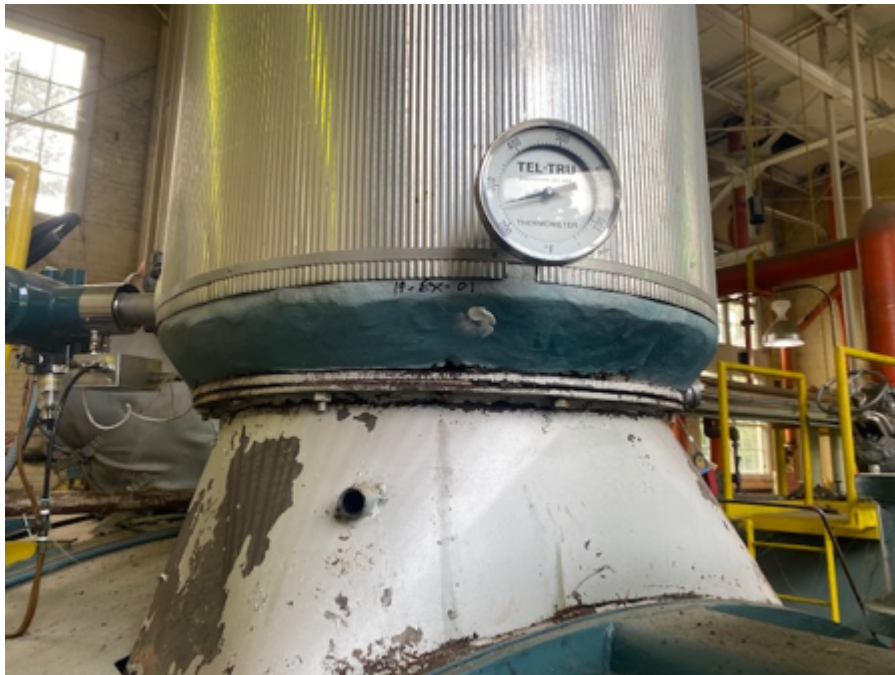
20. Metal Clad Boiler Exhaust Stack (HM #20)
