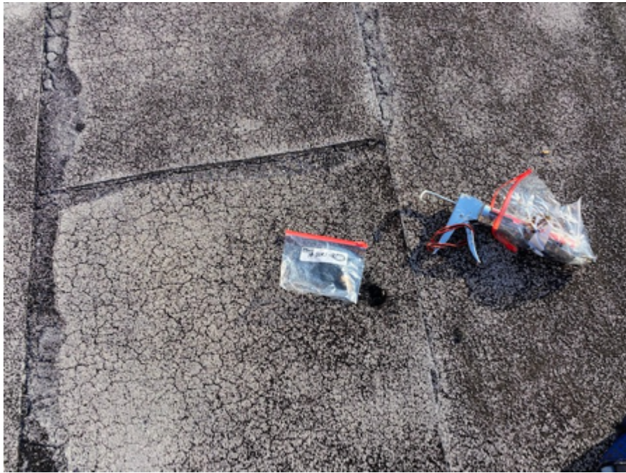
27. Built-Up Roof, Tar and Insulation (HM #27)
