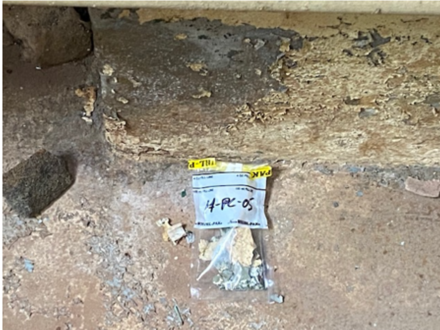
5. Beige/Yellow Paint on Concrete Column, Building 14, Basement, Pump Room (Sample #14-PC-05)
