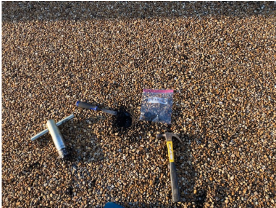
26. Built-Up Roof, Tar and Gravel (HM #26)
