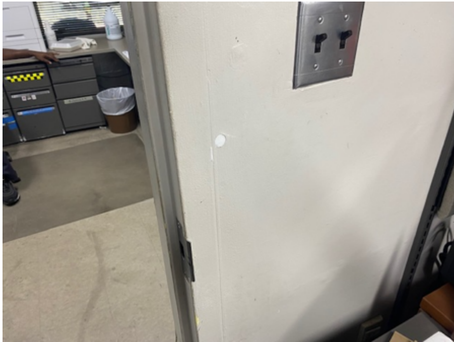
7. Drywall and Drywall Joint Compound (HM #7)
