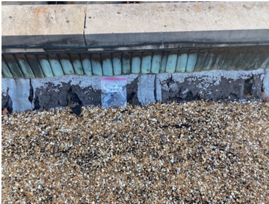
28. Gray Shingle Type Roof Flashing (HM #28)
