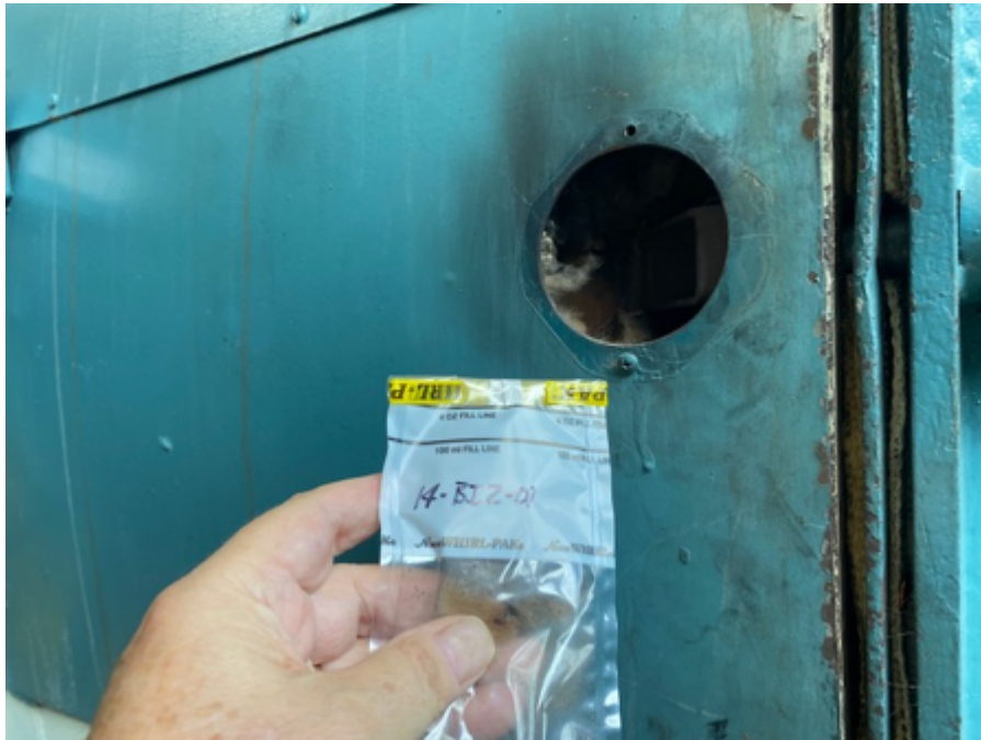
9. Boiler Insulation, Glass Fiber Type (HM #9)
