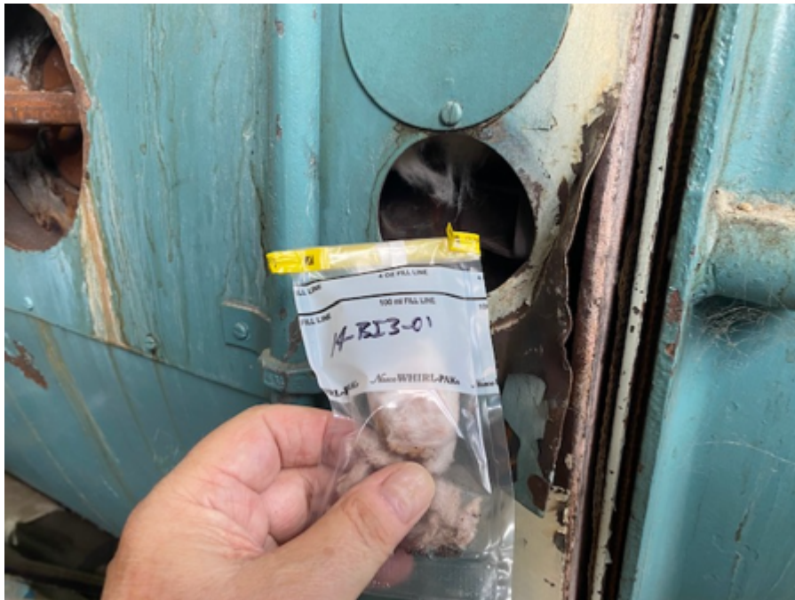
10. Boiler Insulation, Glass Fiber Type (HM #10)
