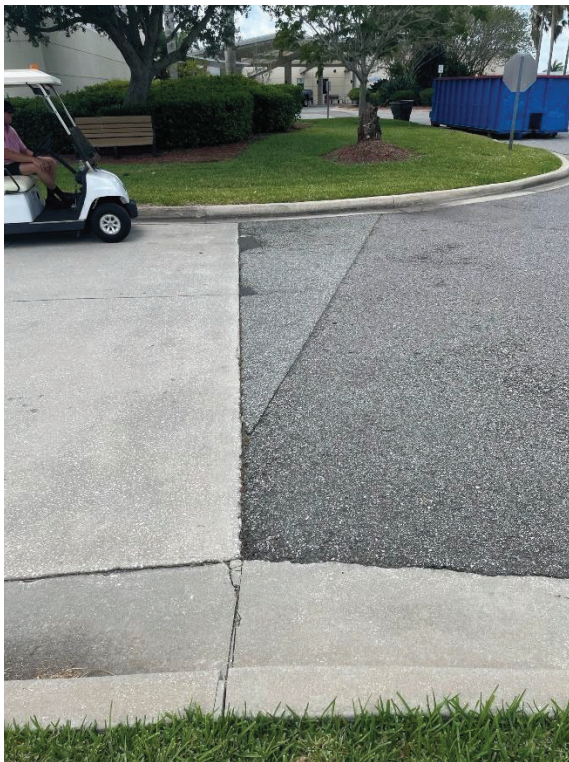
Figure 5: Asphalt-Conc transition repair area
