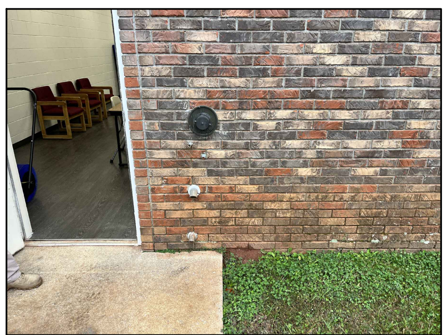
1 EX. FIRE DEPT. CONNECTION (2002 ADDITION) NOT TO SCALE
