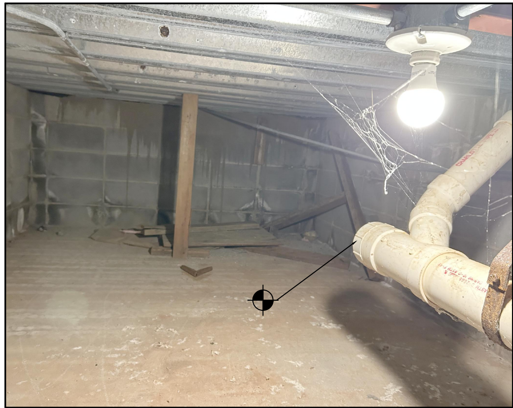
4 EX. WASTE CLEANOUT IN CRAWL SPACE NOT TO SCALE
