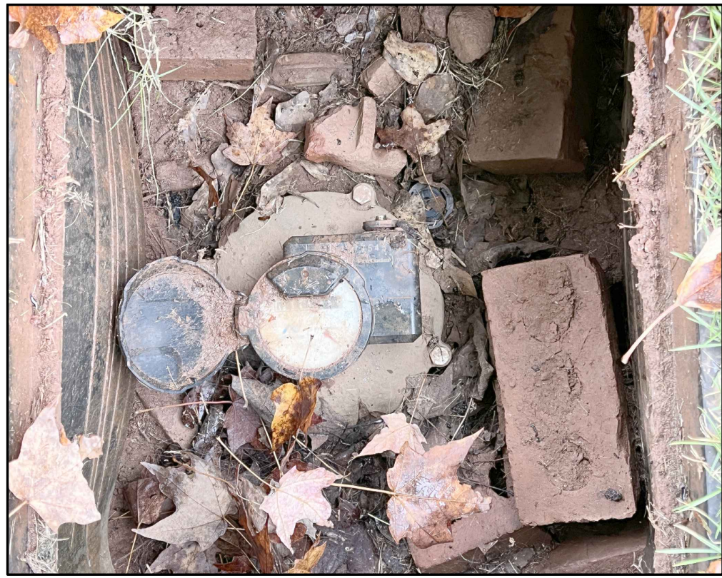
7 EX. WATER METER BOX NOT TO SCALE
