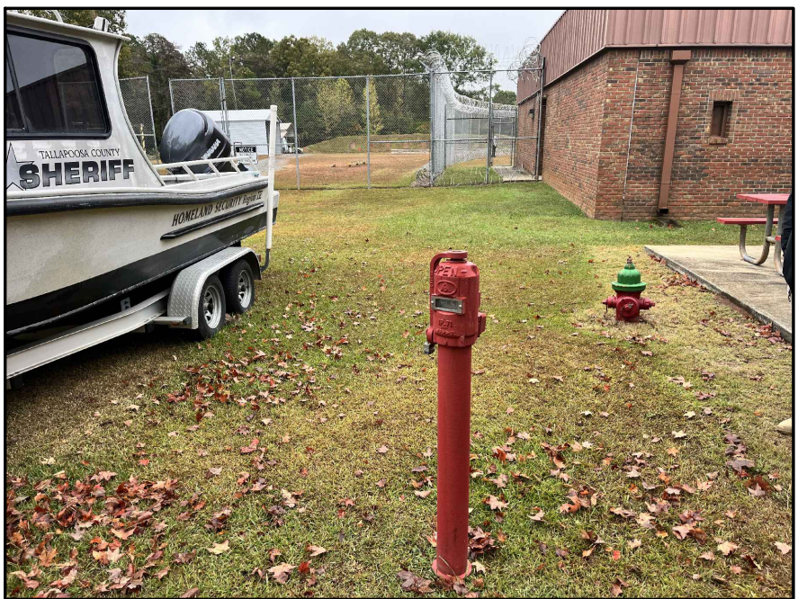
5 EX. POST INDICATOR VALVE NOT TO SCALE
