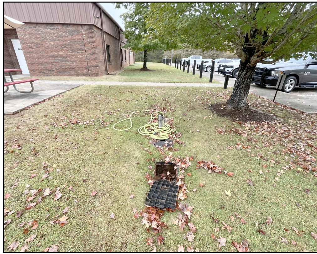
6 EX. WATER METER BOX NOT TO SCALE
