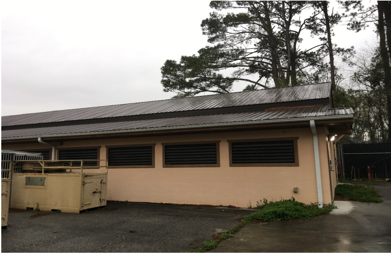
Plate 1: The subject property consists of an approximately 9,000-square foot Working Dog Kennel and associated veterinarian spaces located at the Hunter Army Airfield in Savannah, Georgia. Above is the area where kennels are located.
