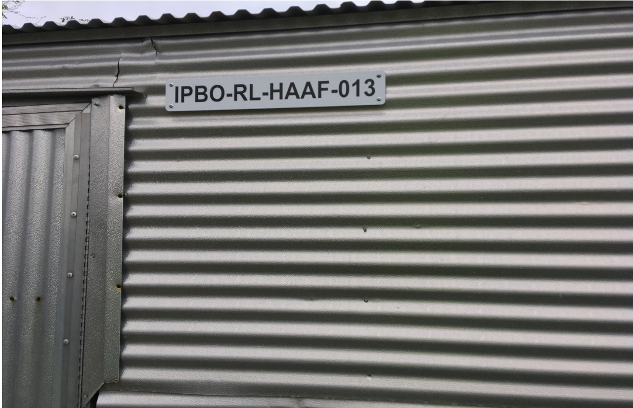
Plate 2: The subject property consists of an additional two steel corrugated metal storage units not operated by the Working Dog Kennel personnel.
